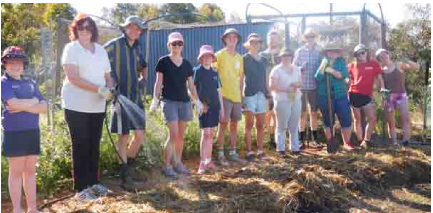
The 2017 'A Different Way' crew, having just finished constructing a garden bed. (That's a garden hose spraying the water ...)
